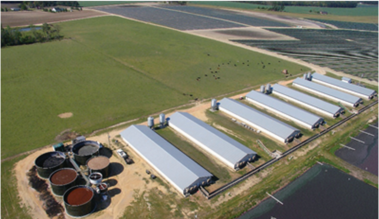
Figure 1. Aerial picture of waste treatment system and barns. It treated all the manure flushed from seven barns with 735 pigs each.
